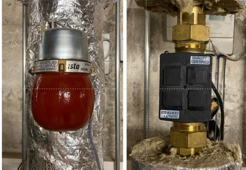
Fig. 17: Old impeller counter (left) and new smart meter (right) for heat consumption measurement
