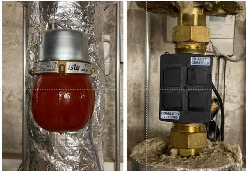
Figure 20: Old impeller meter (left) and new smart meter (right) for heat consumption measurement (Source: CEN)
